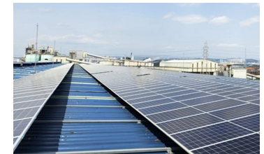
▲ Solar Panels installed on the NP2 Line
